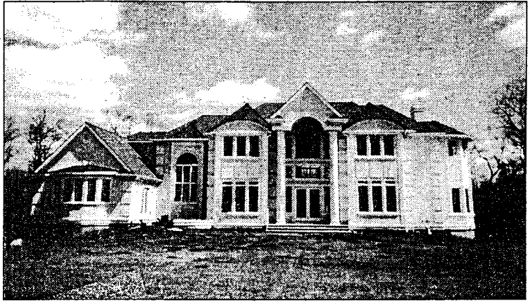
Byron-Hill homes are now under construction in Colts Neck, Marlboro and Holmdel.
