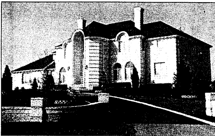
Four Columns will include 21 country estates, such as this Na-nuet design, on large home sites.
